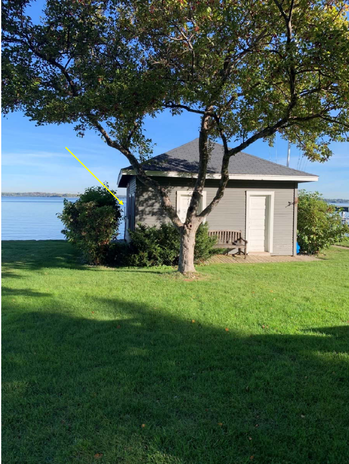
View of boathouse with corner of dock structure slightly visible behind (2022)
